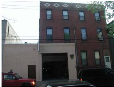
Existing Garage Entrance
