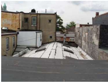
Existing Garage Roof
