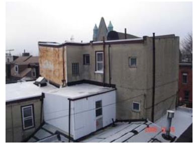
View of Existing Bldgs From Roof
