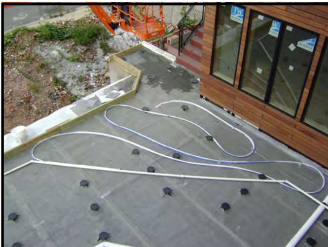
(16) Drip Irrigation System
