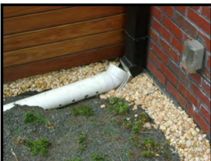
(5) Perforated PVC Pipe
